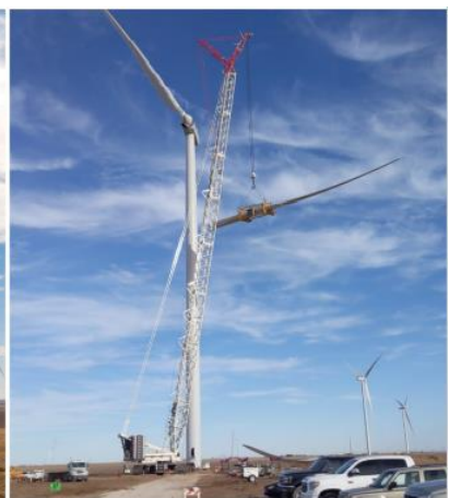
Each turbine has three 199-foot aerodynamic blades designed for maximum efficiency.
