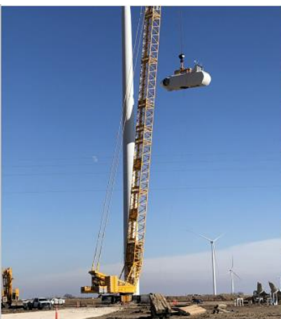
A nacelle is set on top of the towers. The nacelle houses the generator and control systems that work together to convert wind power into electricity.
