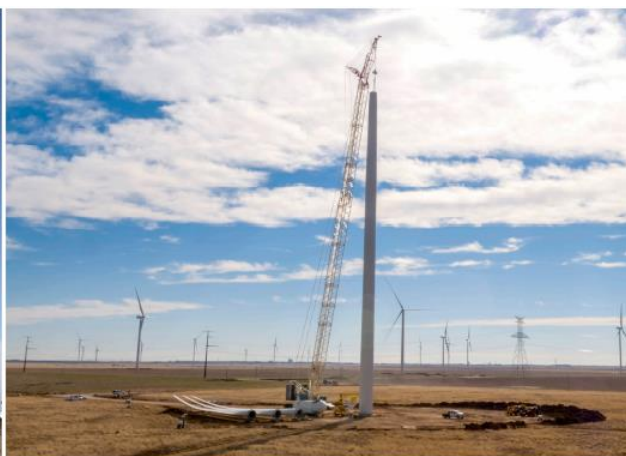
Three sections of towers are set on top of a concrete foundation, standing over 300 feet tall. The final turbine height reaches approximately 499 feet high (at the tip of blade).
